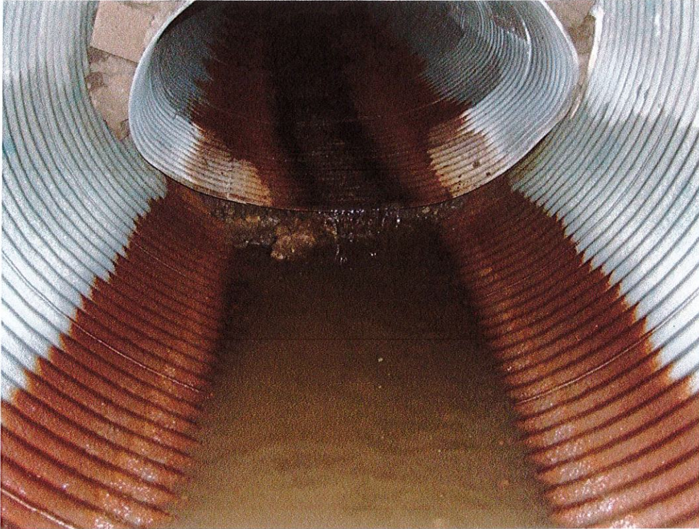
Photo 15. Transition between section 3 and 4 looking north
