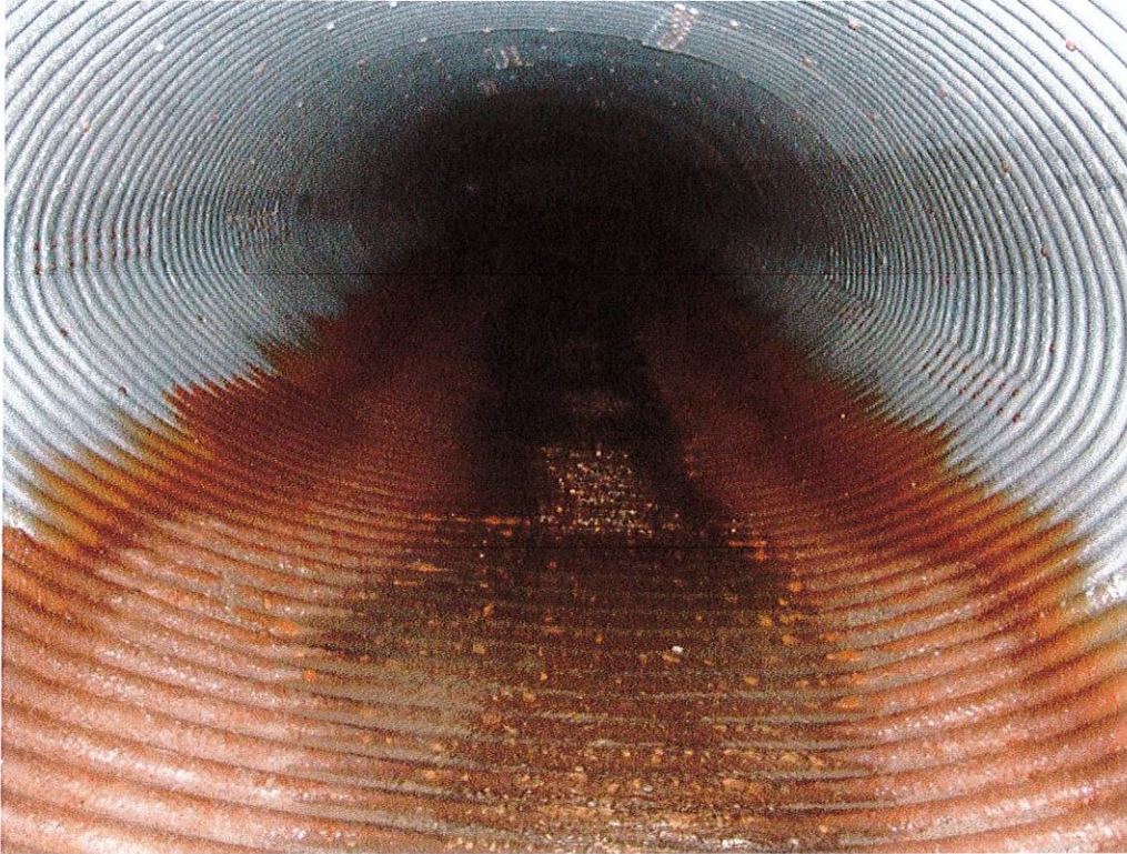
Photo 13. Section 3 barrel looking south
