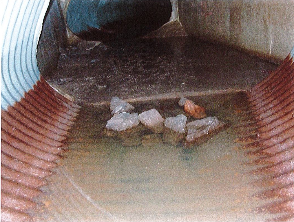
Photo 9. Inlet of section 2 looking south
