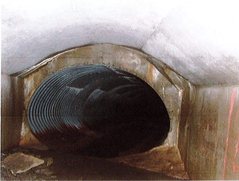
Photo 11. Outlet of section 2 looking south
