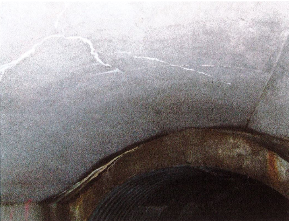
Photo 10. Narrow cracks and light efflorescence in barrel soffit
